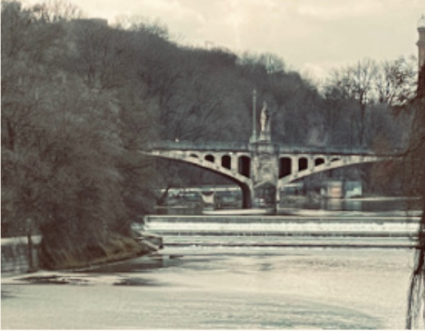
Figure 4. Bridge over the river Isar in Munich/E.Budde
